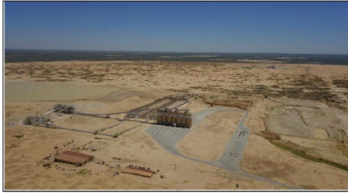
Figure 8.3: Kermit Plant with Truck Loadouts
