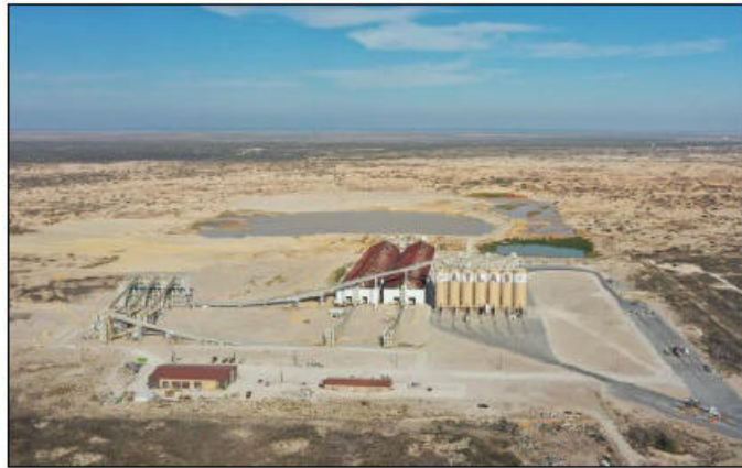
Figure 8.4: Monahans Plant with Truck Loadouts
