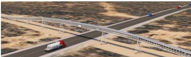
Dune Express Proppant Logistics Infrastructure
