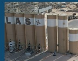
Silos currently going up
